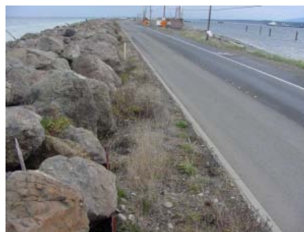
Figure 2: Corps Revetment on North (Strait) side of Ediz Hook
