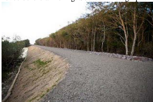
Photo 4 - Levee after armoring July 2010. Source: Photographer Rob Casey
